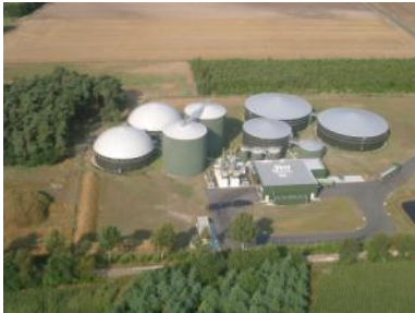
Central Biogas Plant
