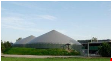
Kitchen Waste Digestion
