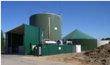
Energy Crop Biogas Plant
