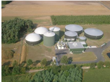
Central Biogas Plant
