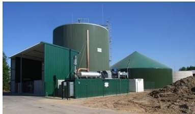
Energy Crop Biogas Plant
