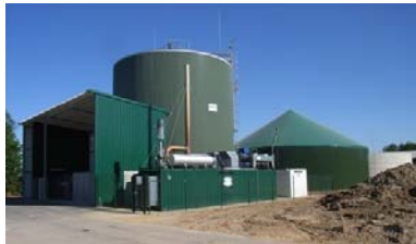
Energy Crop Biogas Plant
