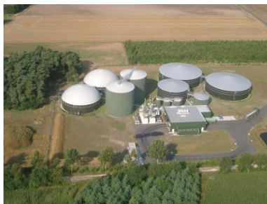
Central Biogas Plant
